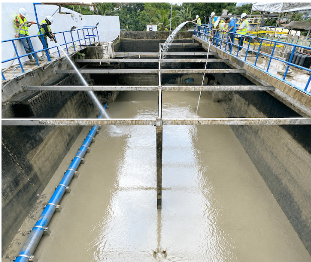
MPBW personnel conduct maintenance and cleaning of the raw water tank at Water Treatment Plant 2, removing accumulated sludge to improve water flow through the facility's filters and help increase water production.
